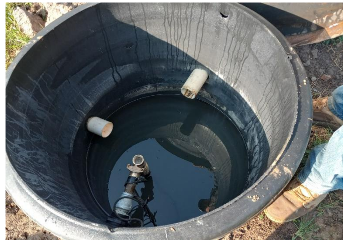
Spring water inlet structure for the Twin Creeks BLM Allotment's livestock and wildlife watering project.
